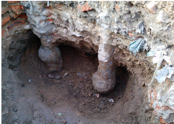
Figure 4. Exposed pile sections with local enlargements, shown from two viewpoints.
