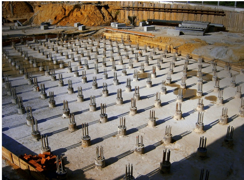
Figure 7. A pile field before construction of the superstructure.
