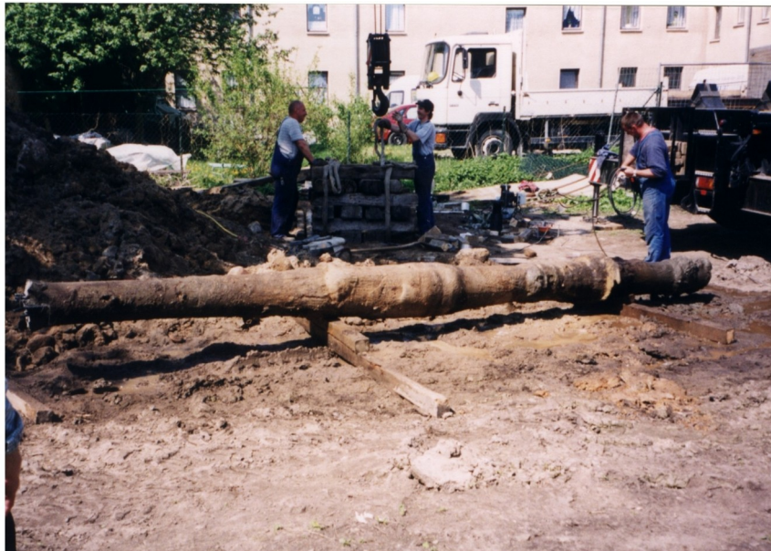
Figure 6. An extracted pile with enlargements along its shaft.
