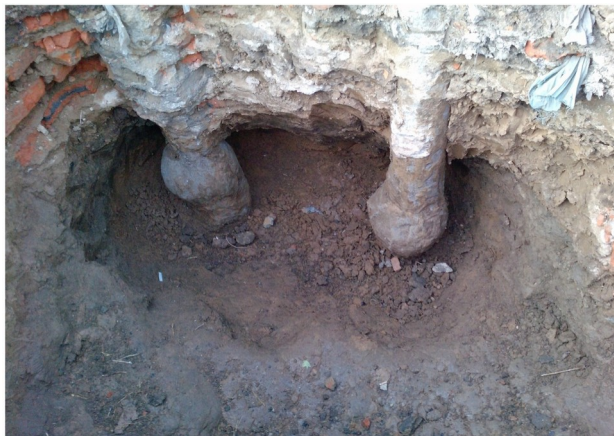
Figure 4. Exposed pile sections with local enlargements, shown from two viewpoints.
